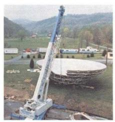
The 62-foot diameter dish rests on an area of lawn where it was constructed. A short time later, the 120-ton crane hegan the lift.
