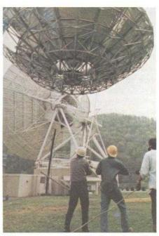
Workers use rope to steady the load as dish rises into the air.
