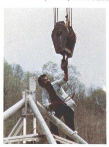
Once dish was in place, the quadripod structure was lifted from the ground and set inside it. Here a worker prepares to attach crane hook to the top of quadripod.
