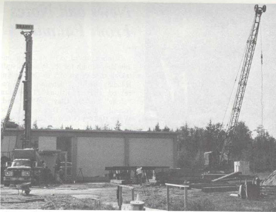
Construction for the new antenna has already made some inroads at Andover.
