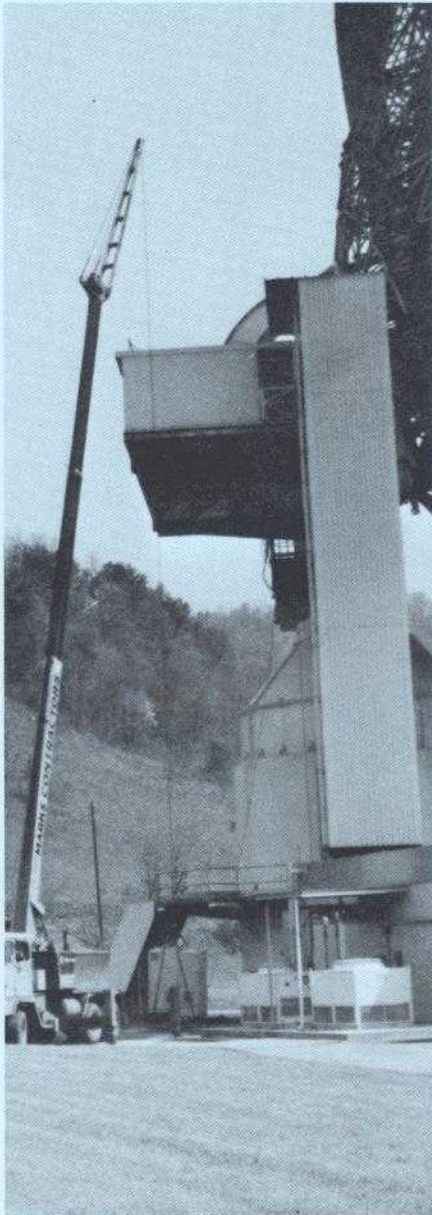
The high-powered amplifiers are put in place by crane.
