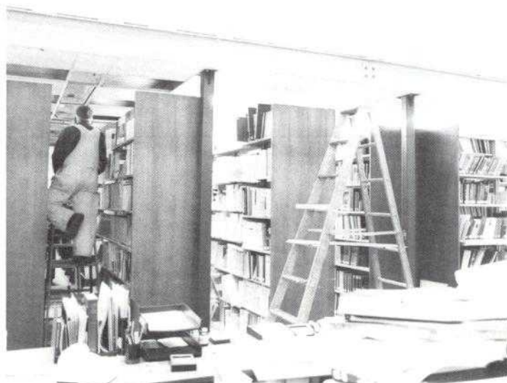
A. Fleming about to install the east ceiling section.
