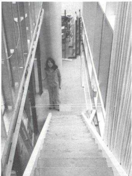
Librarian Liu surveys completion of first phase of construction.
